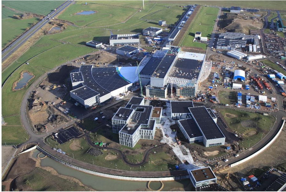
Figure 1: Aerial view of the ESS facility (January 2021). Image: Perry Nordeng/ESS.
