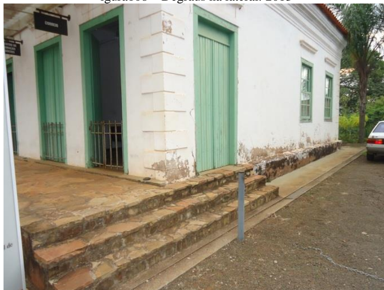
figura108 – Degraus na lateral. 2013
