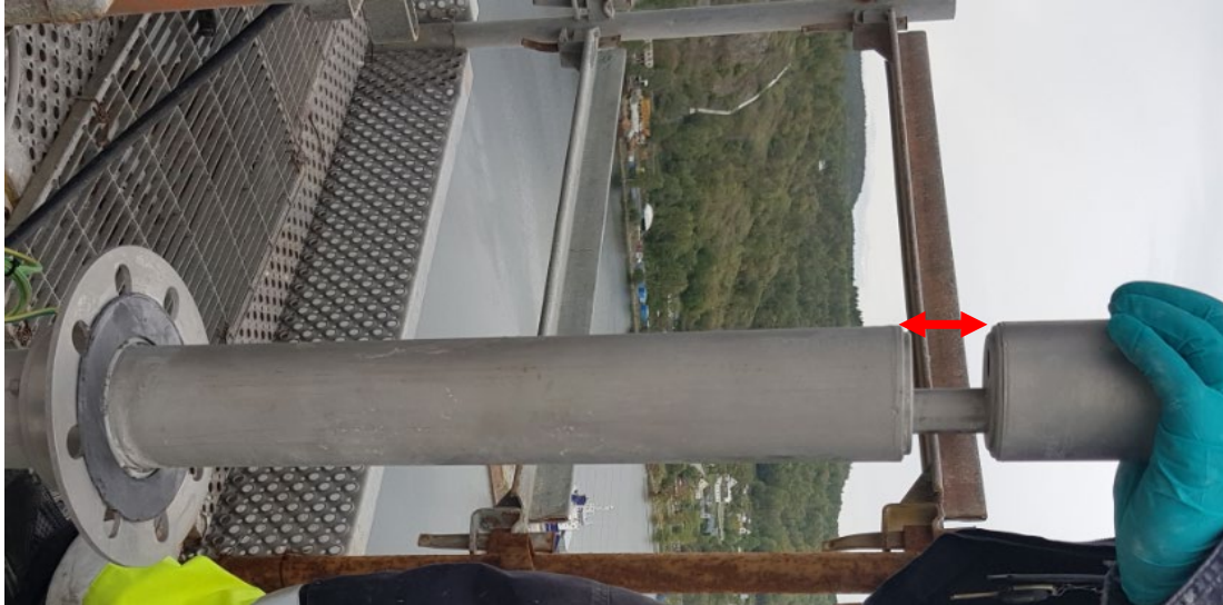
Figure 11 OSA probe which one goes inside the stack.
