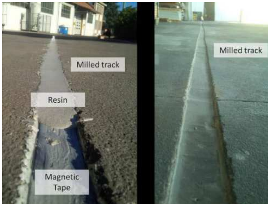
Figure 13: Preparation for magnetic navigation [5]
