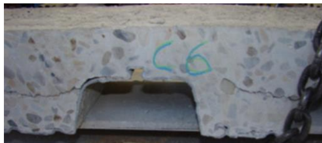
Fig. 19: Cracking: composite slab [66]
