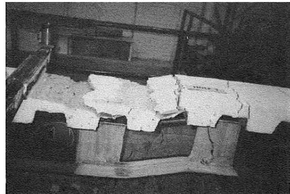
(b) Failure at web opening with high moment-shear ratio
