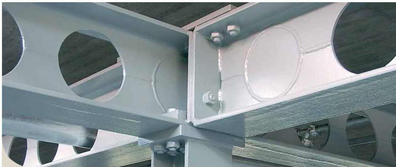
Fig. 2: Filled openings at support [1]
