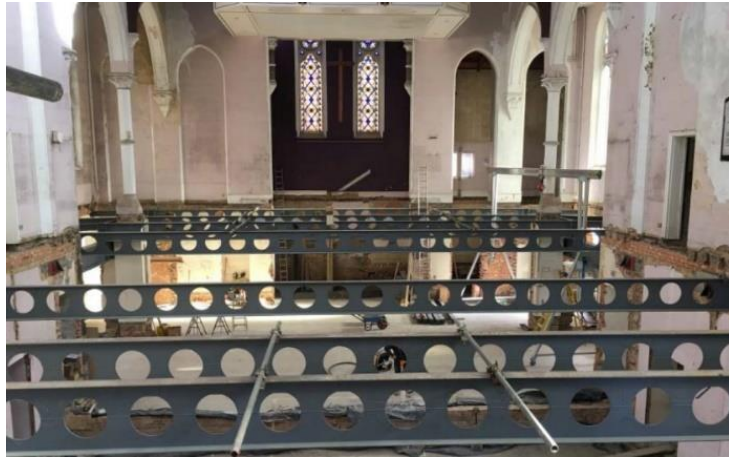
Fig. 2: Restoration of Royal Vale Church [14]
