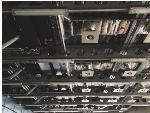
Fig. 5: Ducts passage for the integration of services [14]
