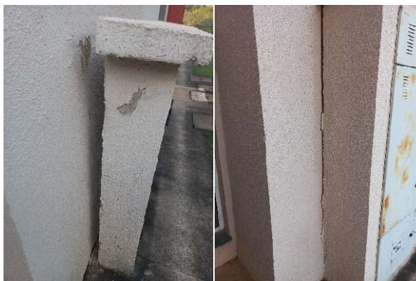
Figura 28: Recalque
