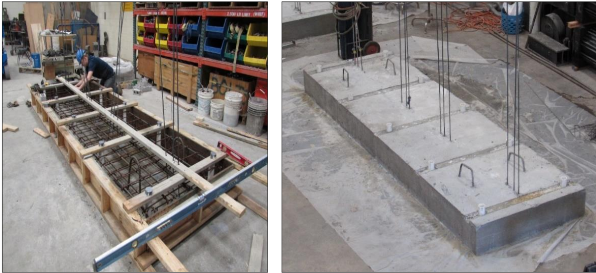
Figure 27: Foundation of the walls.
