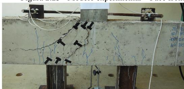
(a) BA_{s,sold}0 : face frontal - fissuras na ruptura
