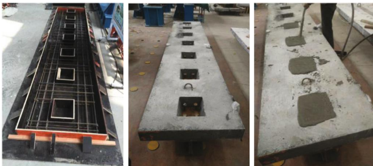
(a) Manufacturing of slab with shear pockets
