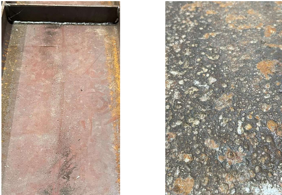
(a) Surface of non-corroded beam
