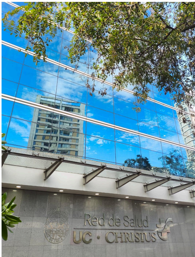
Figura 3- Fachada do hospital UC Christus, Santiago, Chile.
