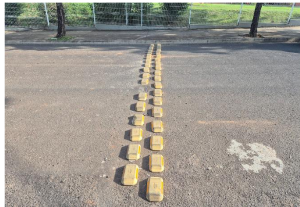
(n) Tachão 2 - lateral
