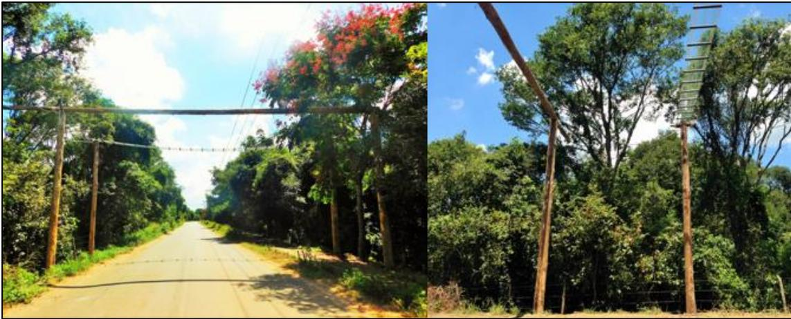
Figure 2: Two canopy bridge designs: a rope bridge and a wood pole bridge,
