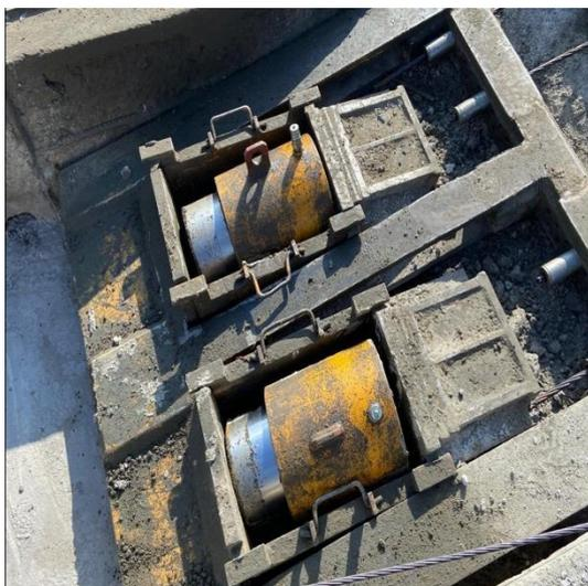
**Figura 4-18 Cordoalhas desprotedidas, verificado com o cilindro com curso mínimo**
