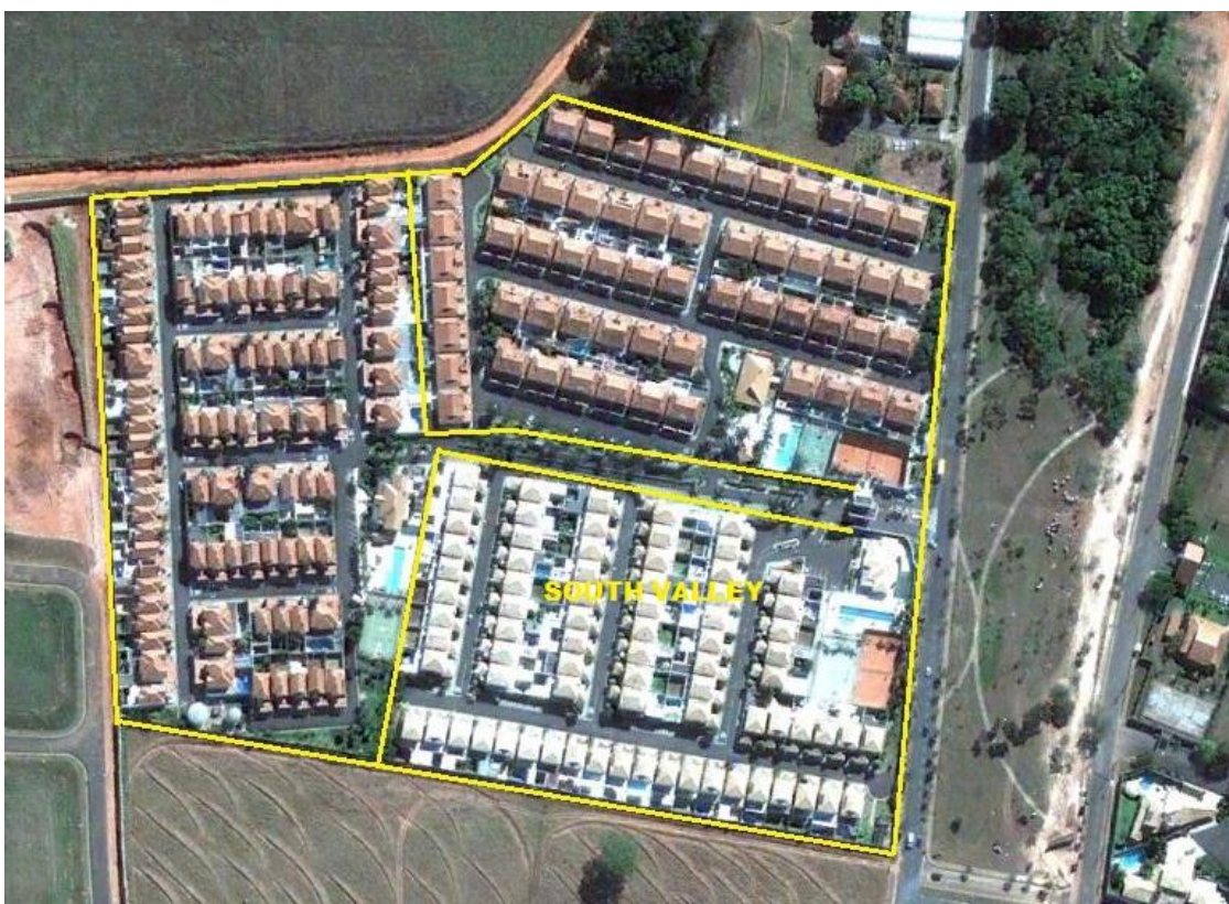
Figura 65 – Vista do Condomínio Green Village – South Valley
