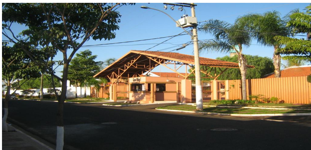
Figura 36 – Portal de entrada do Green Village I
