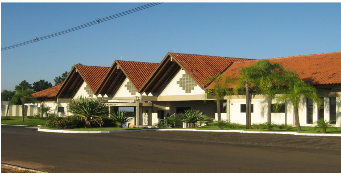
Figura 35 – Portal de entrada do Village de La Montagne
