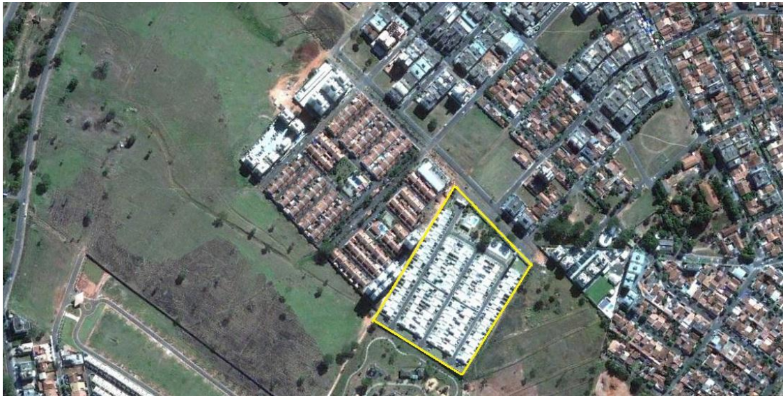
Figura 74 – Vista geral do Condomínio Green Village III
