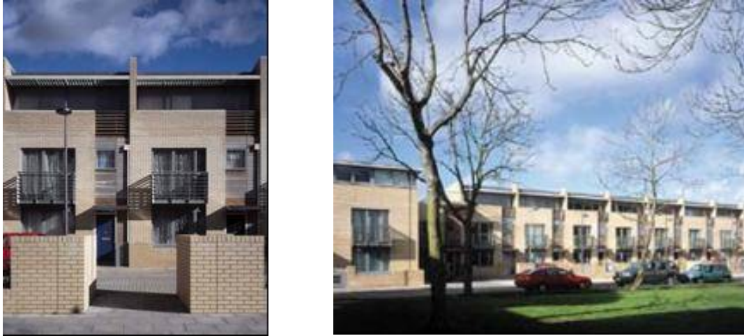
Figura 3-18 Project participants: Lambeth Housing, Ujima Housing Association, Presentation Housing Association, Family Housing Association (Angell Town Estate Management Board, Angell Town Community Project, Government Office for London) with Burrell Foley Fischer, Anne Thorne Architects, Greenhill Jenner, Mode 1 Architects, solarcentury and other.
