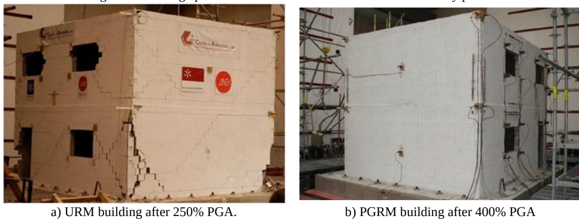
Figure 22: Damage patterns observed at the ultimate seismic intensity phase.
