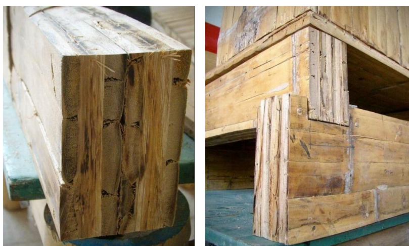
Figura 74 – Crushed Bamboo Beams
