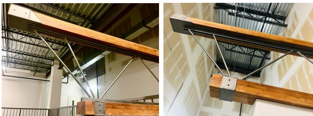
Figura 62 – SEB + Welded Steel Web and Bearing Plate
