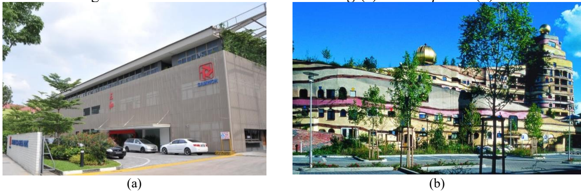
Figura 2.14 – Samwoh Eco-Green Building (a) e Waldspirale (b)
